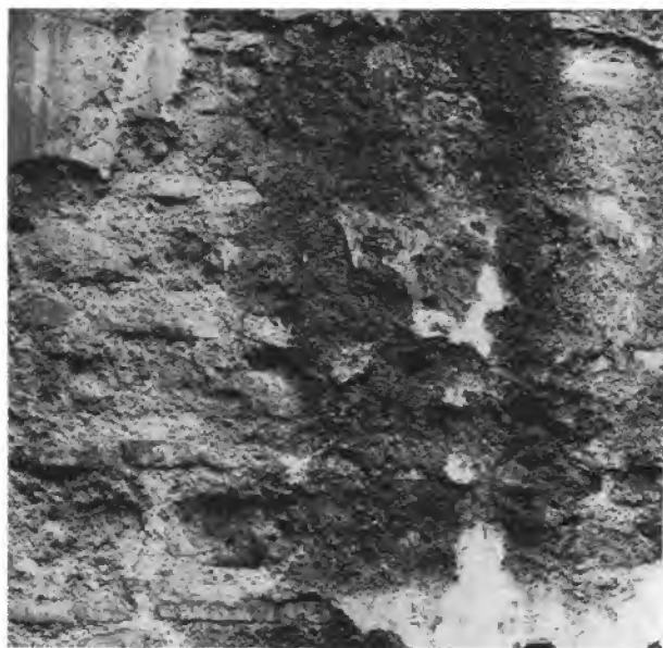
Fig. 147 — S. Lorenzo in Lucina. Opus listatum of apse wall, near right hand shoulder (Photo: Sansaini).
